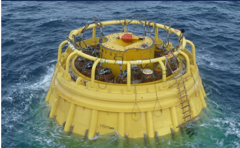
STP buoy/turret pre-ballasting
