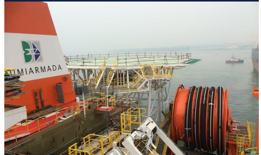
Helideck & loading hose/reel installed
