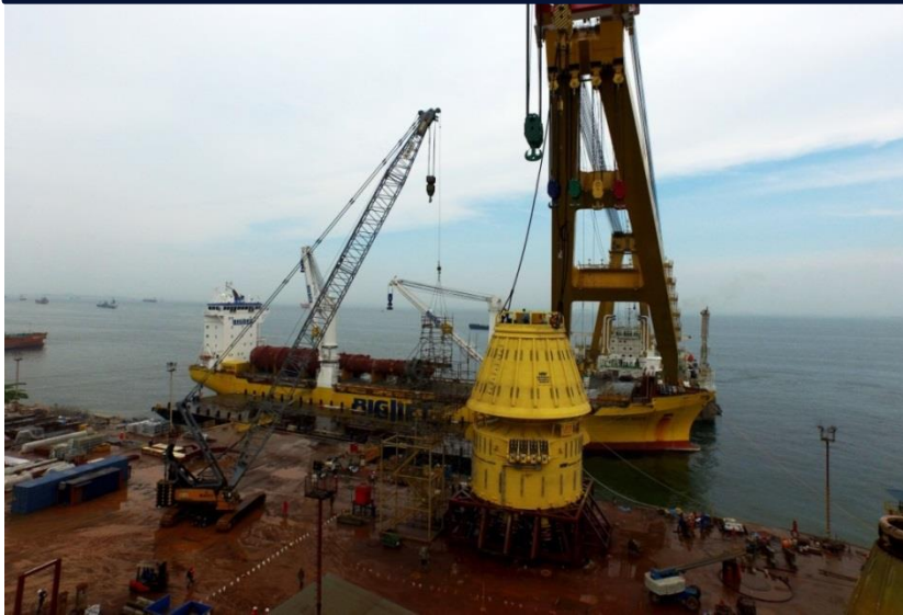
STP buoy/turret pre-ballasting
