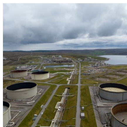
View of Central Avenue Sullom Voe Terminal
