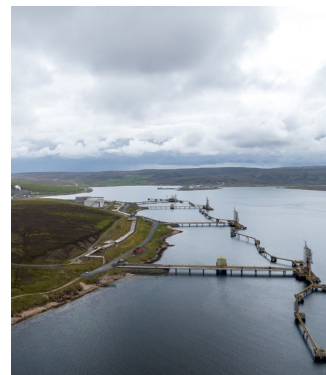
A view across Sullom Voe to the port of Sella Ness showing the four deep-water jetties at SVT
